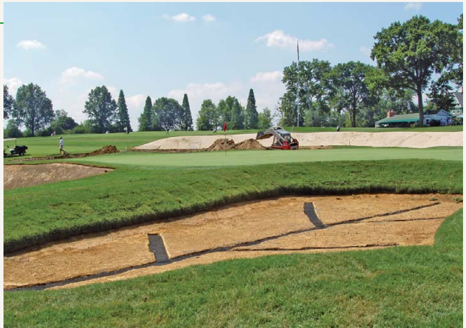
A large portion of the restoration work is targeting the course's 190-plus bunkers
